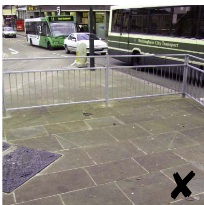
Mount Street - pedestrian safety barrier
