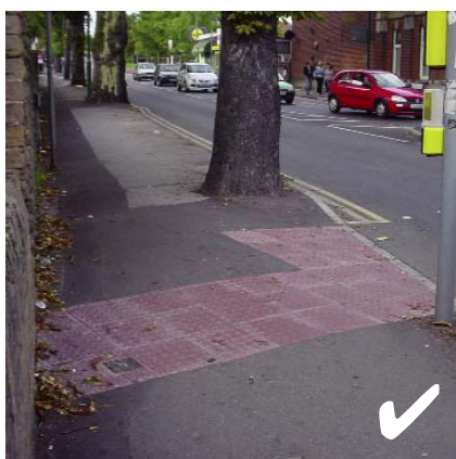
Contrasting tactile paving
