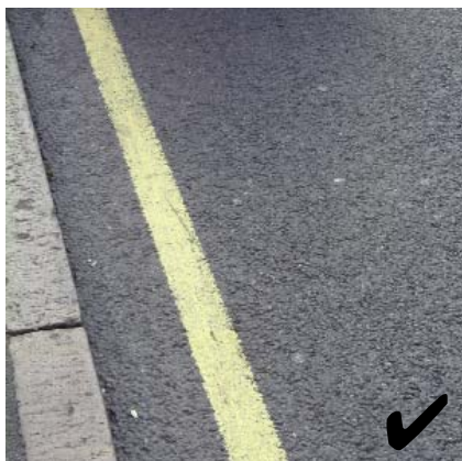
Carlton Road - stone masticated asphalt
