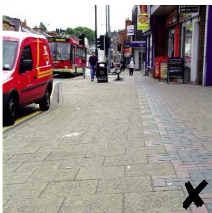
Mansfield Road, Sherwood - small unit paving
