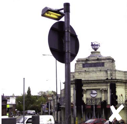
Lower Parliament Street - externally illuminated sign light backwash
