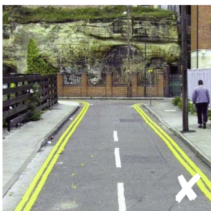
Pemberton Street - intrusive lining
