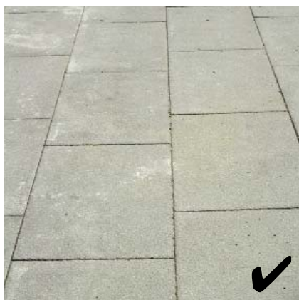
London Road/Victoria Embankment - large rectangular re-inforced slabs
