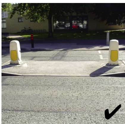
Southchurch Drive - paved splitter island
