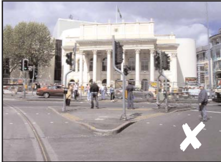
Market Street/Upper Parliament Street - cranked signal poles
