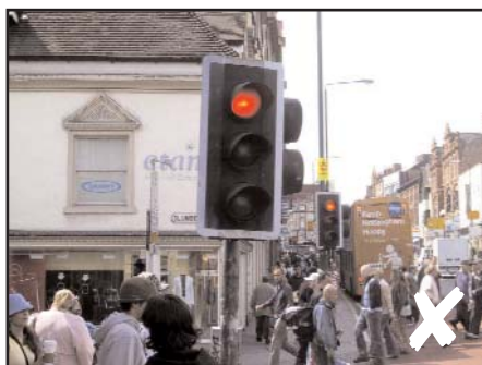
Clumber Street - signal backing boards
