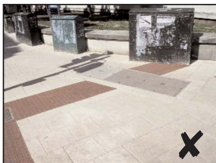
Goldsmith Street/Burton Street - no inset tactiles
