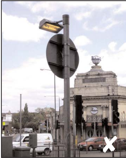
Lower Parliament Street - externally illuminated sign light backwash
