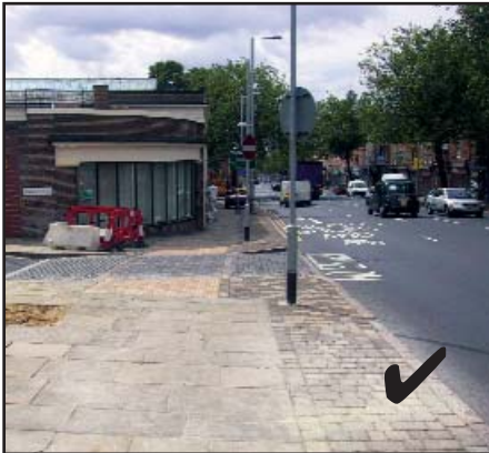
Villa Road - narrowed width speed table (under construction)
