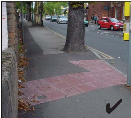
Contrasting tactile paving
